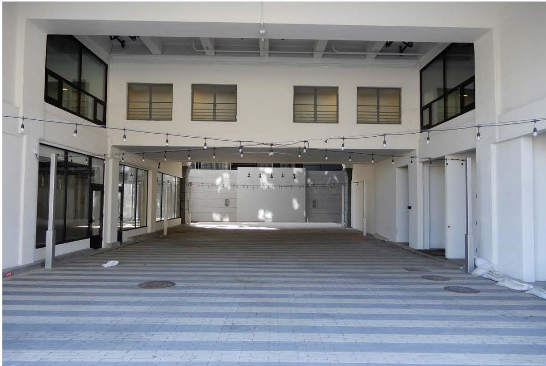
Photo 3 - East elevation, former Pike passthrough, looking west
