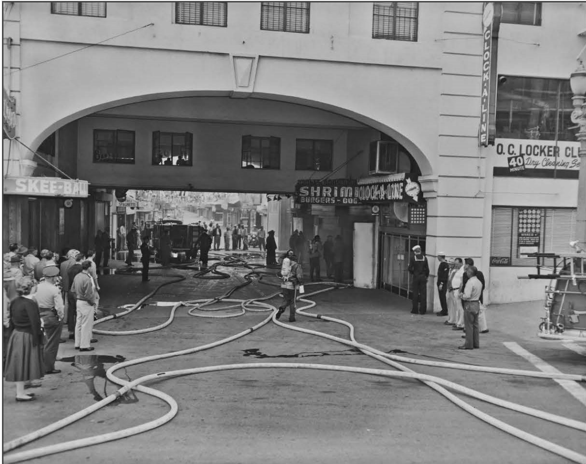
Fig 17. Ocean Center Building showing the building's passthrough. A fire at the Hollywood Bar was extinguished.
