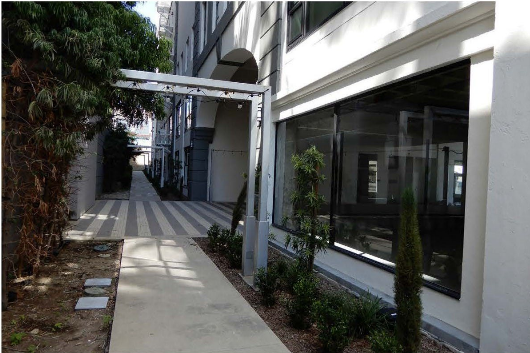
Photo 5 - West elevation and pedestrian alley, looking north
