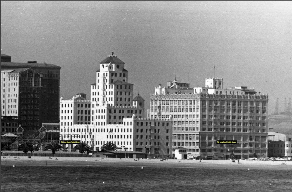
Fig 14. Ocean Center Building and beachfront. Source: Long Beach Public Library Digital Archive, photo 1935
