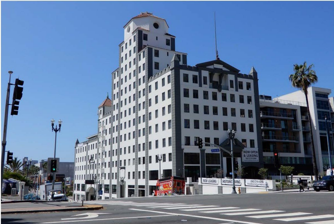
Photo 1 - North and east elevations, looking southwest
