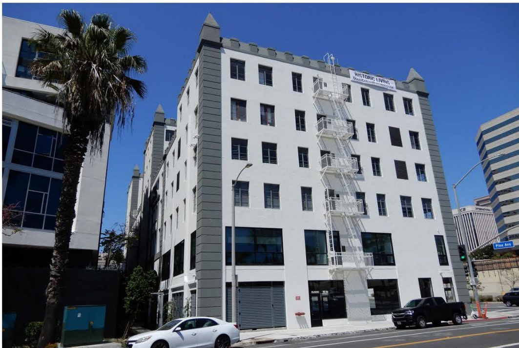
Photo 4 - South elevator, looking northeast
