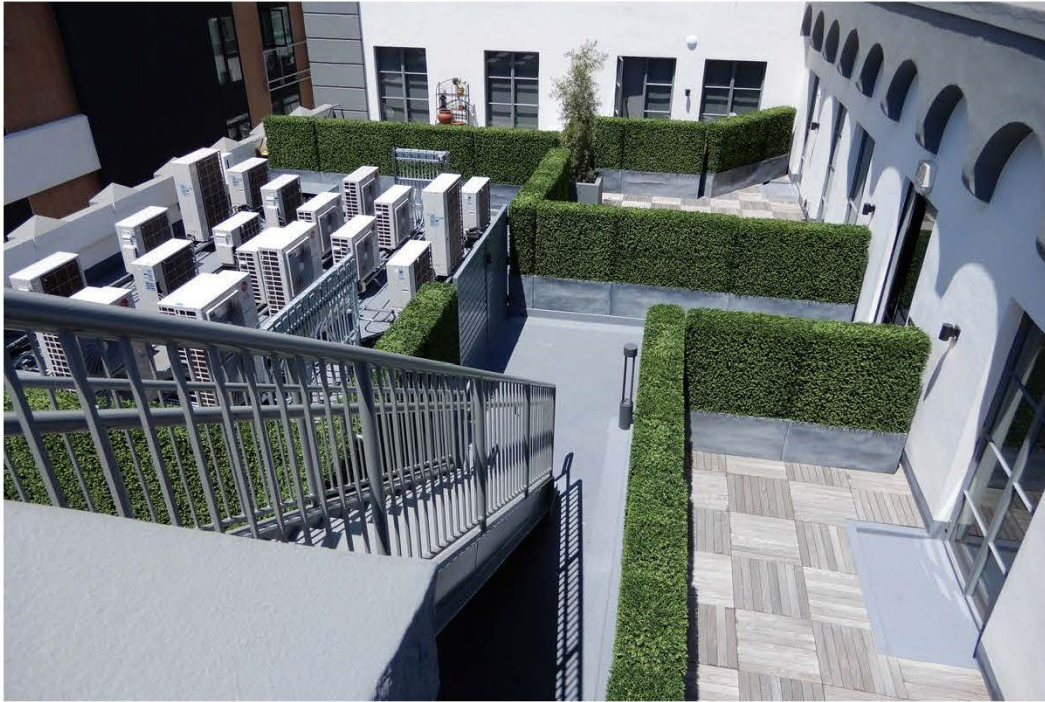
Photo 27 - 5th floor, looking down at 4th floor south light court, looking north
