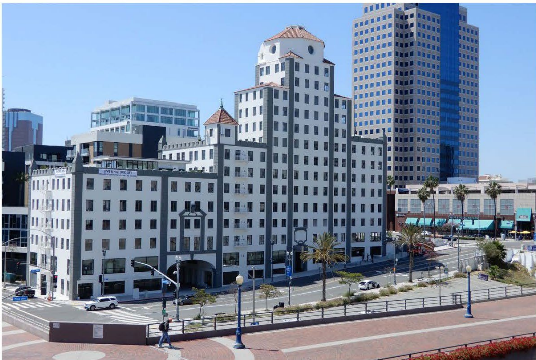
Photo 2 - East elevation, looking northwest
