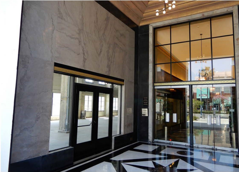
Photo 11 - 1st floor, main entry vestibule, looking southeast
