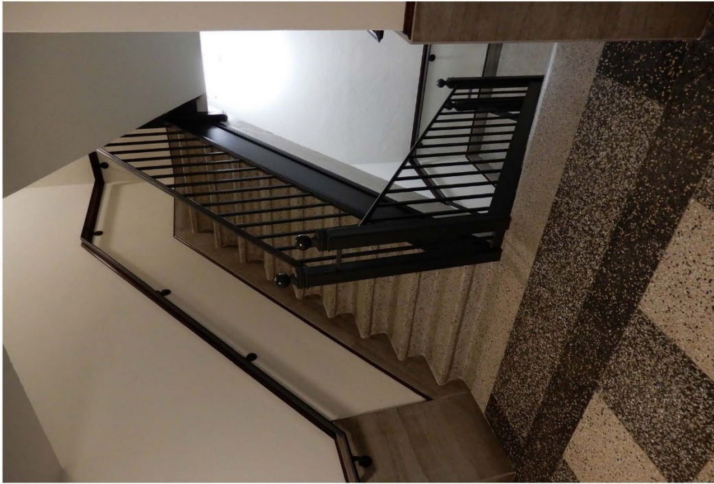
Photo 23 - 5th floor, south stairs, looking southwest
